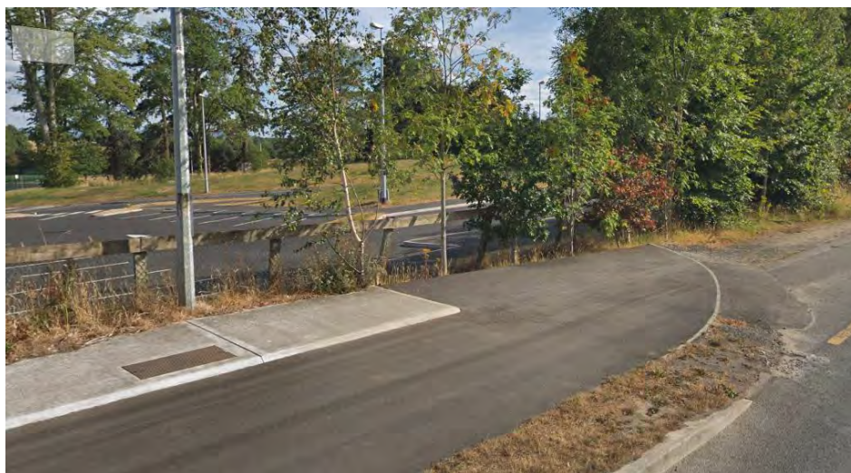
Figure 4.29: Barrier to School Cycle Lane on R448
