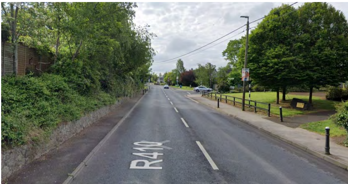
Figure 6.22: Photo of Blessington Road
