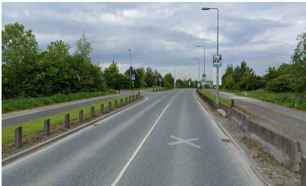
Figure 6.36: Photo of Southern Ring Road
