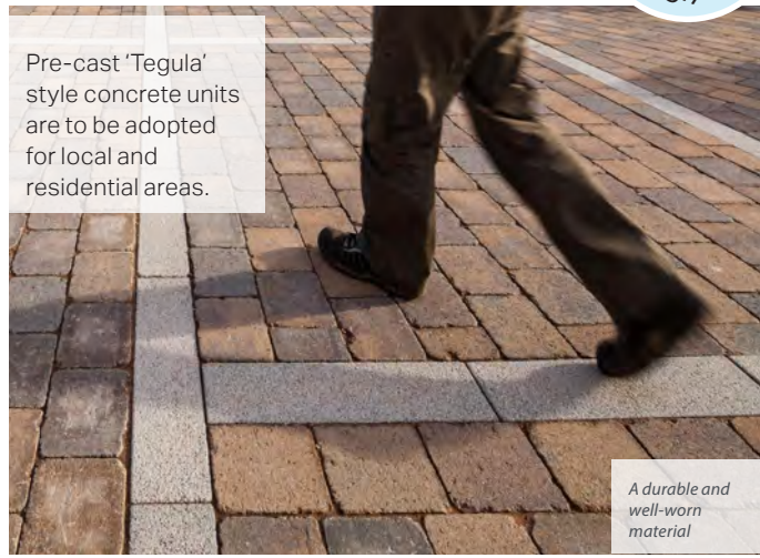
A mix of exposed granite aggregates, set into pre-cast concrete paving units, offer high-quality and durable finishes
