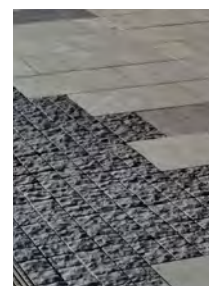
Clean transition between cropped granite (left) and feature paving.
