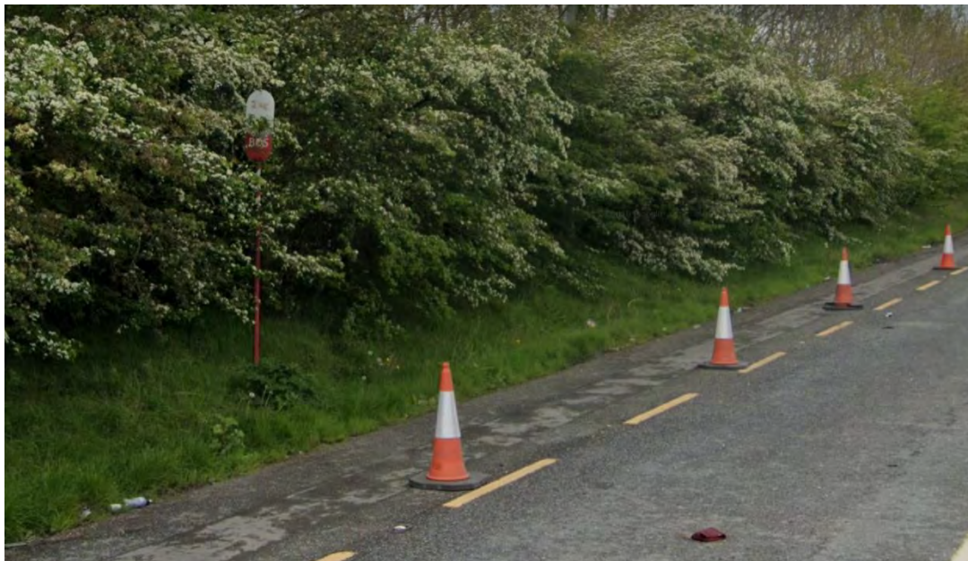
Figure 4.4: Example of Poor Bus Stop Infrastructure on R445
